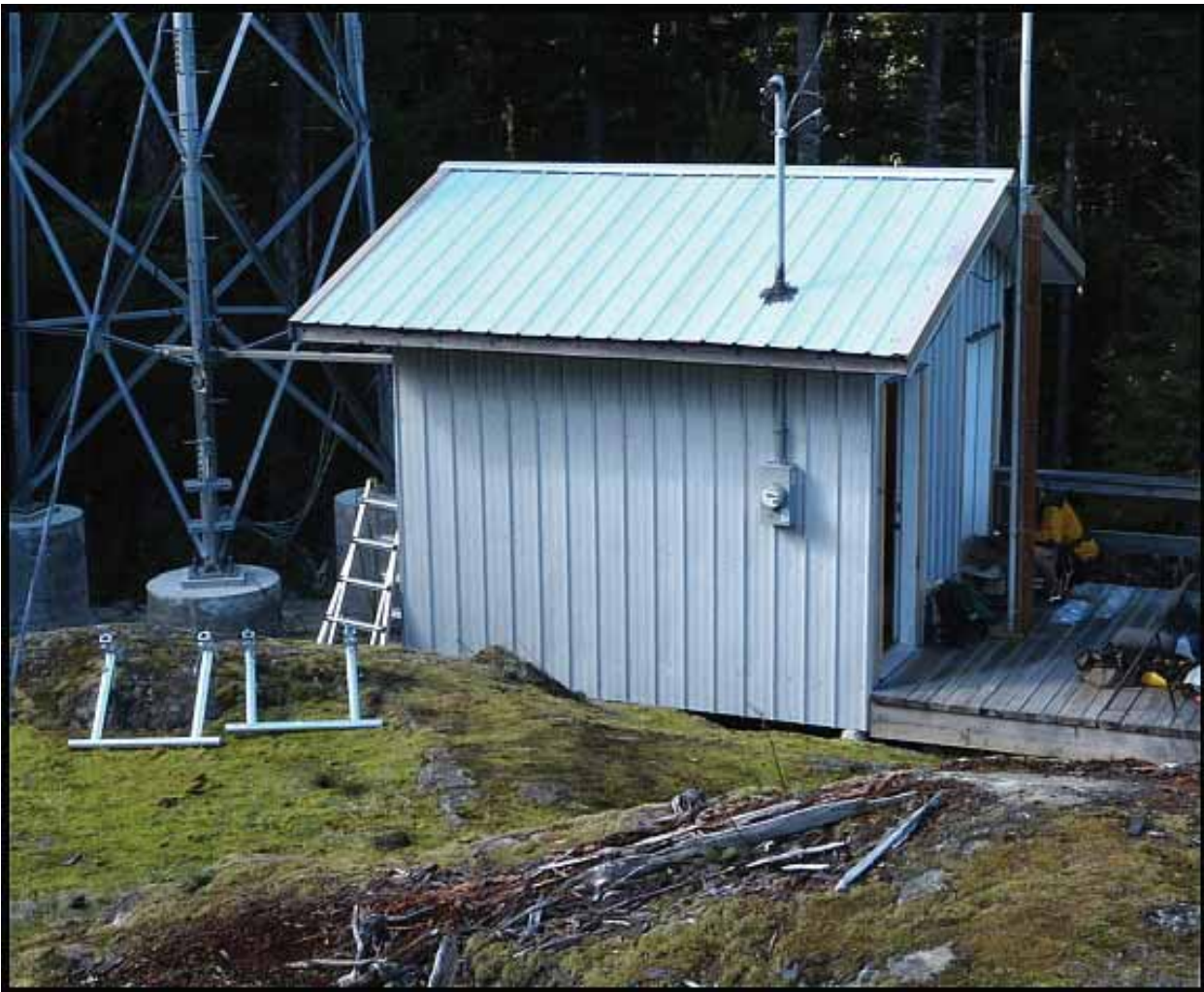
GBIS - The Mount Pocahontas shed at the base of the new tower.
