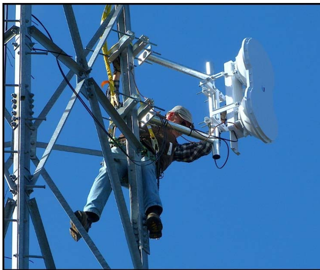
Alan Davis installing the new backhaul dish on the Pocahontas Tower.
