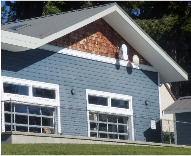
Original (on right) and new backhaul dishes at Sunshine Coast Health Centre, south of Powell River.
