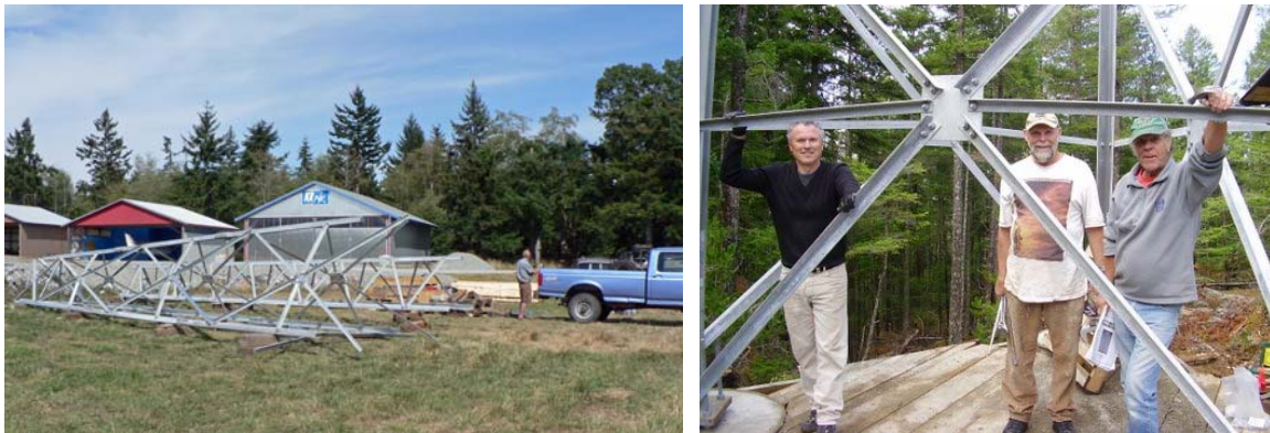
The tower was partially assembled at the Gillies Bay airport; the bottom section was assembled on site.
