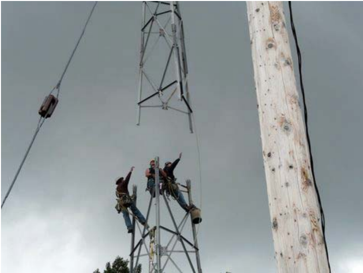
The Prestige crew on the tower as each section arrives by helicopter.
