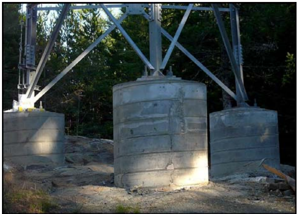
Over 200 bags of special concrete were used on the base, plus special grout on each leg.
