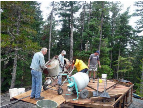
Volunteers mix the concrete for the base; on the right an anchor bolt is pull-tested.
