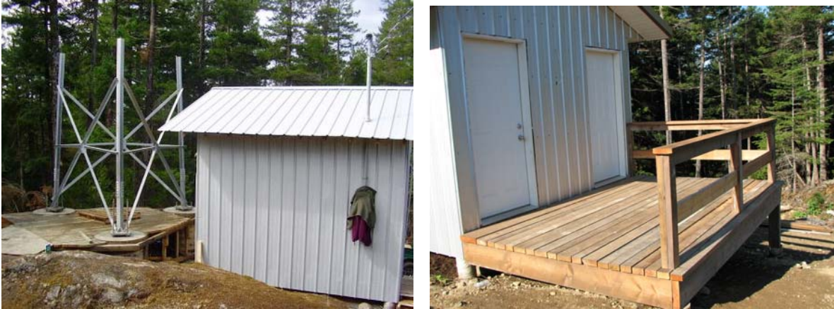
The GBIS building on Pocahontas contains routers and the PEP emergency repeater equipment.
