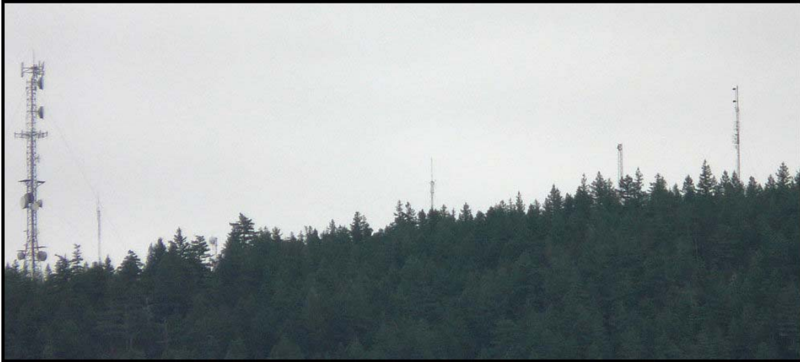
If you have a good line-of-sight you should be able to see 6 towers on Pocahontas. They are (L to R) BC Hydro, Canadian Electronics Corp, Telus (low down), DFO/RCMP, GBIS and CBC.
