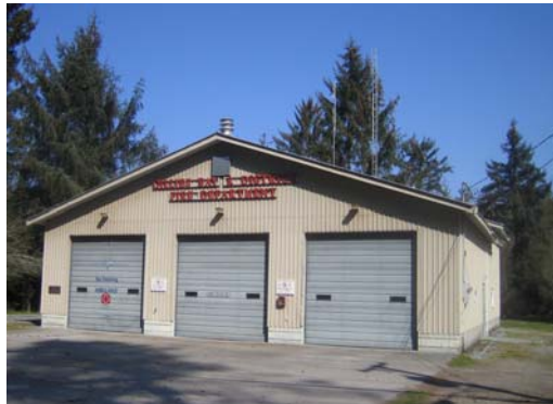
Gillies Bay Fire Hall
